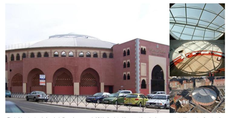
The bullring structure in Aranda de Duero is composed of 36 inclined steel frames set in a circular arrangement with an outer diameter of 80.00m and an inner diameter of 46.00m.
